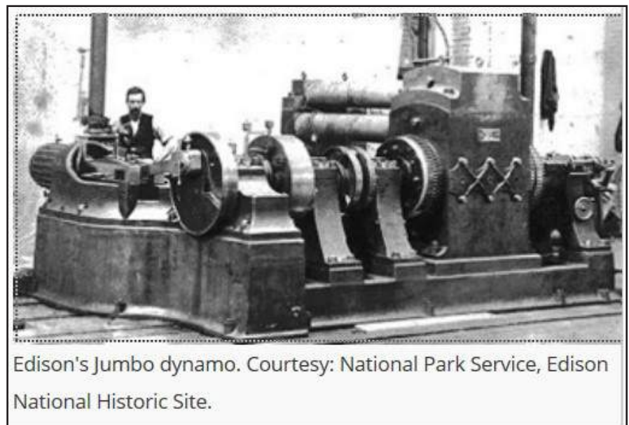
Figure 02 : Edison's Jumbo dynamo
